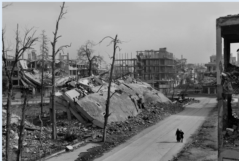
Figure 6: The severe damage caused by the ISIS attacks in Iraq and Syria 33
